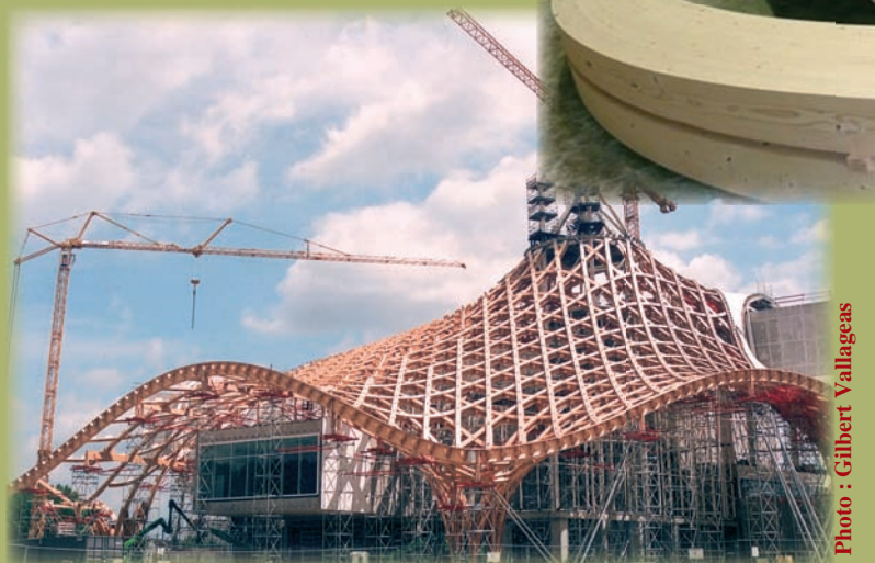
Centre Pompidou Metz
